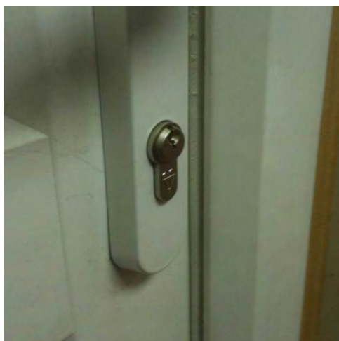
Example of a correctly fitted cylinder
